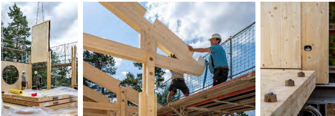
Image 5: Details of the construction: infill exterior walls, load-bearing skeleton und reversible connection of wall elements with the CLT slab with cone adapters. Photo: Eckhart Matthäus
