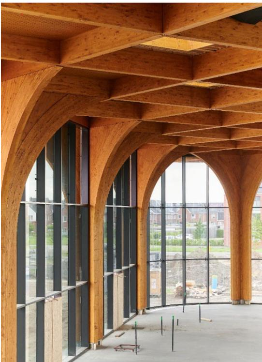
Picture 5: Diagonal grid of cross-shaped curved trusses
