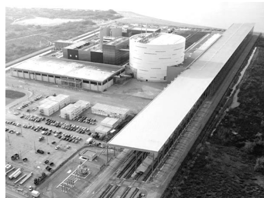
Figure 2: Aerial view of the construction
