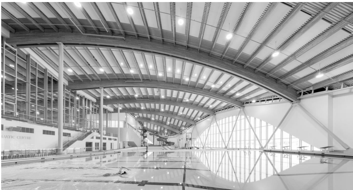
Figure 5: Interior Over Aquatic Centre - Image GEC
