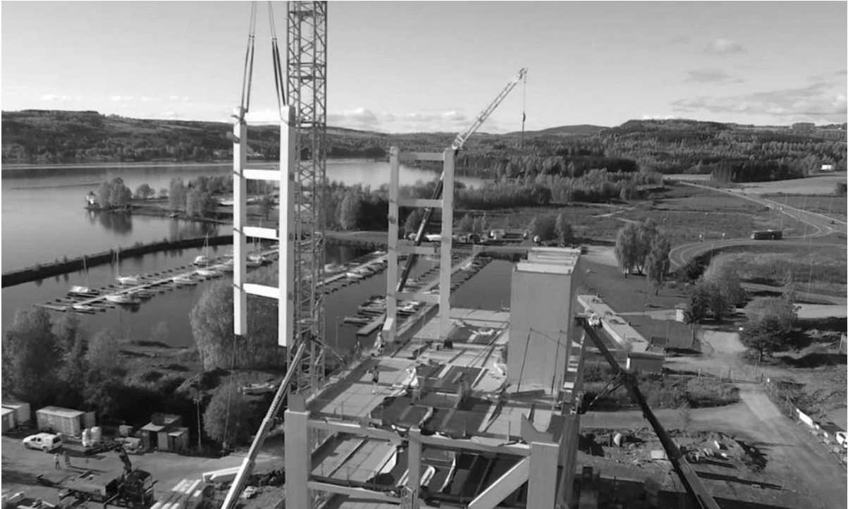
Figure 16: Installation of large glulam structures preassembled on site
