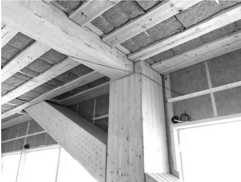
Figure 3: Accelerometers were installed directly onto structures
