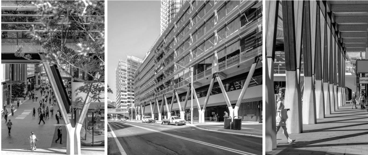
Figure 5 – 7: International House Sydney colonnade with Y columns constructed from solid recycled ironbark hardwood
