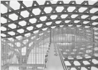
Holz-Gitterschalen Timber Grid Shells
