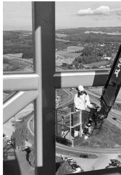
Figure 7: Glulam sections throughout the pergola have rounded edges to reduce the wind load
