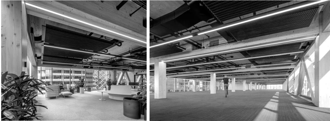
Figure 12 and 13: Exposed timber and expressed services provide the character and interior quality to the workplace
