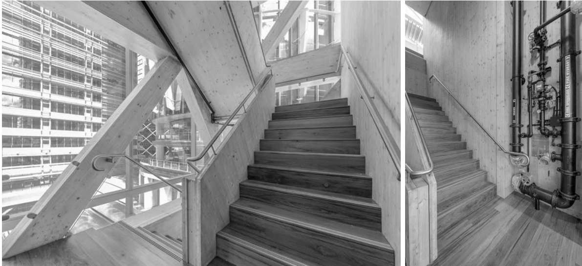
Figure 10 and 11: Internal egress stairs invite use for movement between floors – constructed from CLT and treads and risers lined with recycled hardwood
