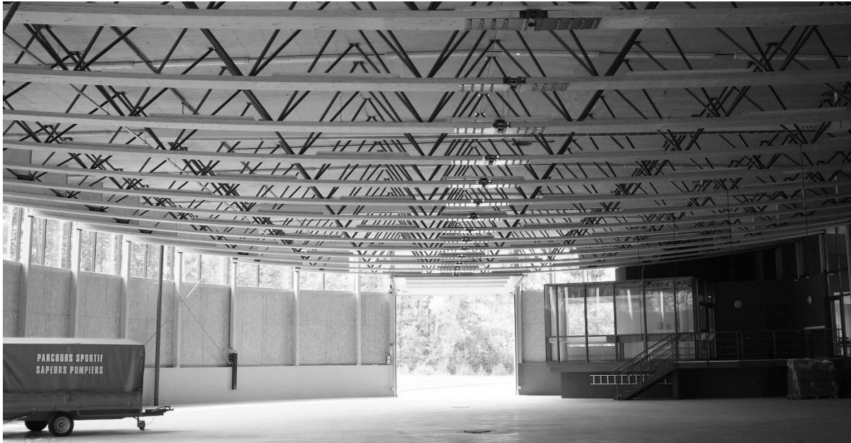
Figure 10: Inside view of the main hall
