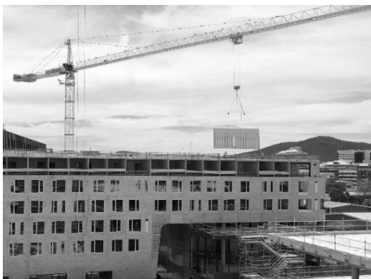
Figure 16: ANU, façade panel lift
