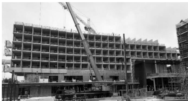
Figure 15: ANU, Student Accommodation CLT
