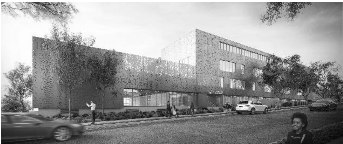
Figure 6: Perforated aluminium façade overlay
