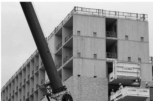
Figure 17: ANU, Student Accommodation façade over CLT
