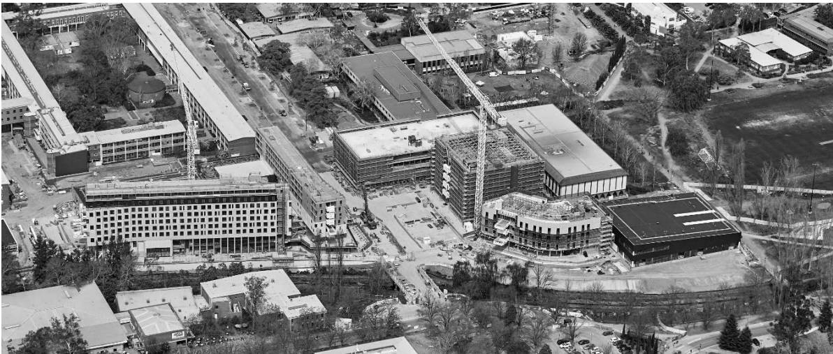
Figure 8: Kambri, ANU development during construction
