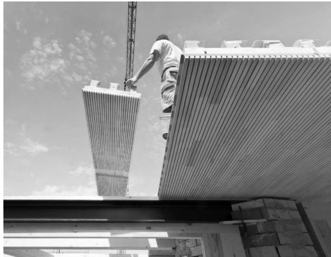
Figure 3: OLA, proposed four storey atrium Figure 4: OLA, Floor slabs with integrated Lignotrend installed
