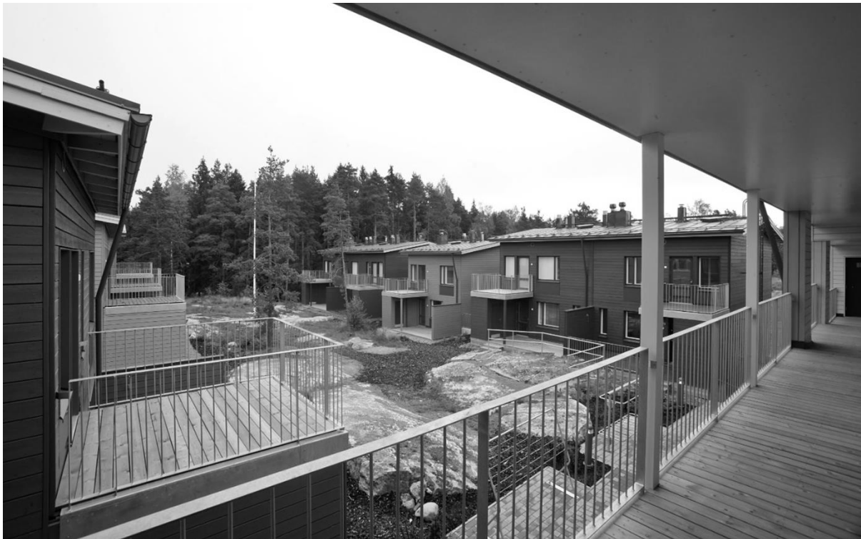
Figure 2: Village-like wooden housing district Wood-Myllypuro will be completed in 2018.
