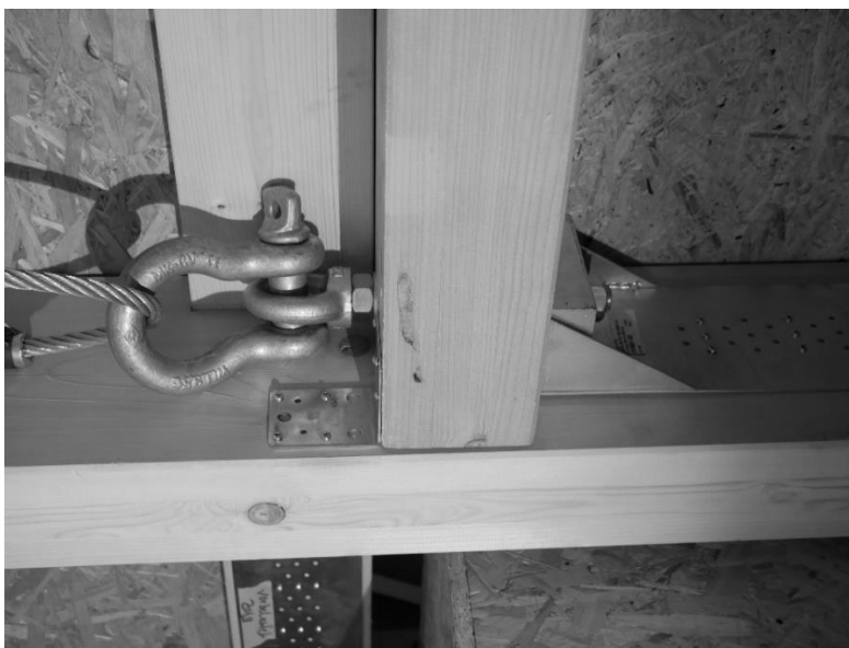
Figure 8: Anchorage on floor slab to pull on the building.
