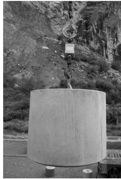
Figure 11: Balance suspended on crane to weigh all pieces set in place.
