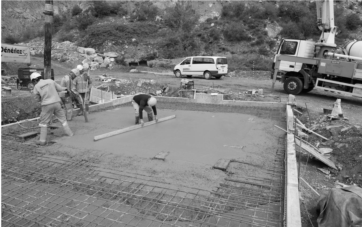
Figure 9: Pouring the concrete of the foundation. Anchorage pieces are already set.
