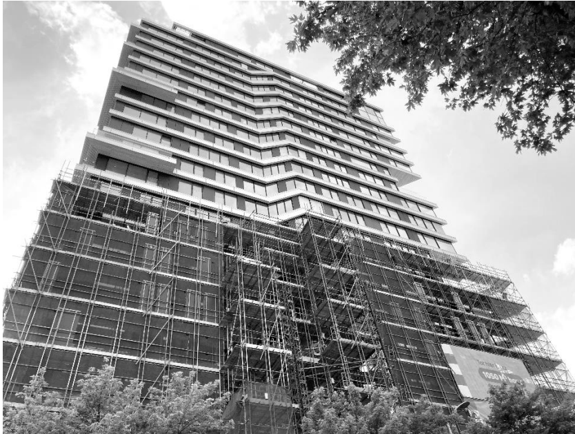
Figure 1: Construction site in July 2021
