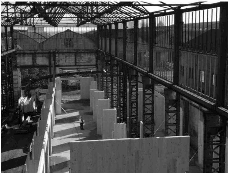
Figure 5: On site installation of the wall panels of the ground floor
