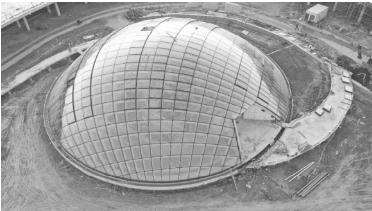
Figure 20: View of the Small Dome with glazing complete
