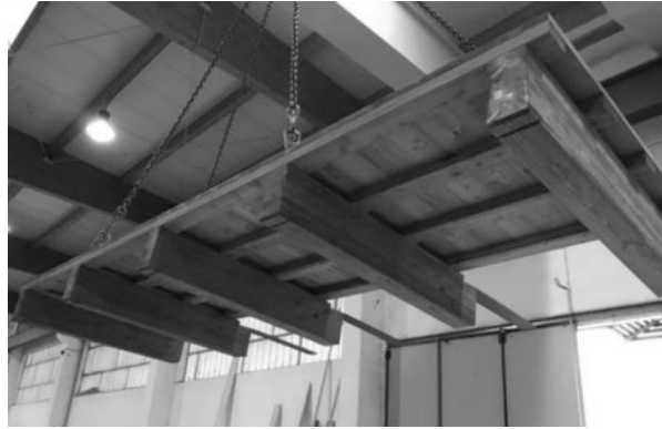
Figure 9: Construction of Xlam balconies in the factory.
