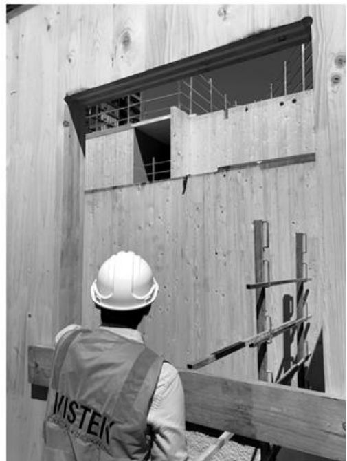
55 Southbank: A 10-storey CLT vertical extension during construction in Melbourne
