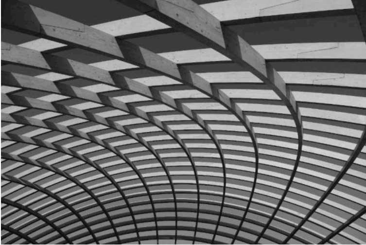
Figure 19: View of the completed glulam in the Small Dome
