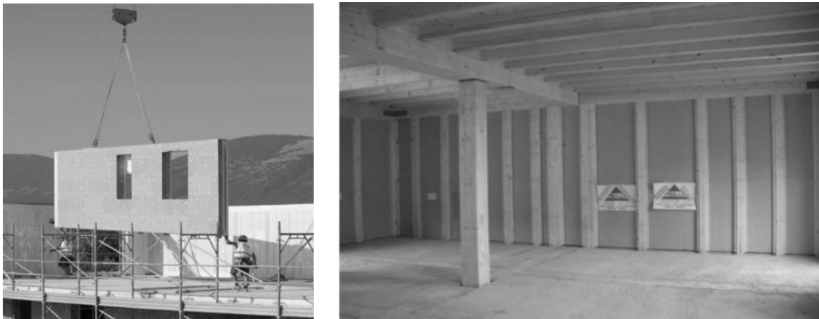
Figure 1+2: Images from the construction site: safety for operators and cleaning site.
