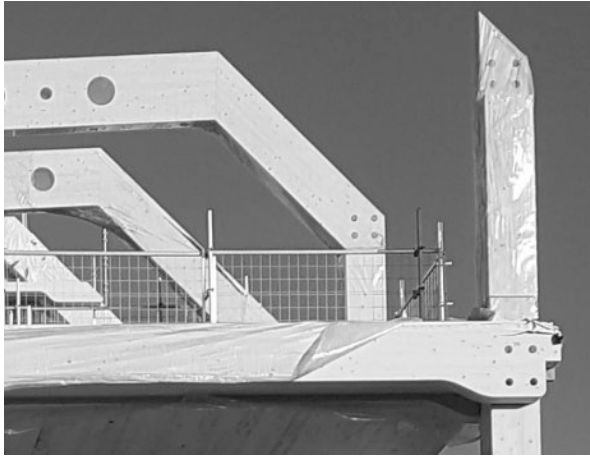
Figure 8: On site picture. Direct timber connection
