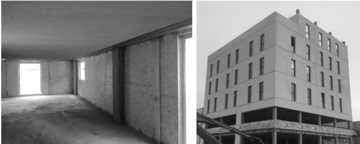
Figure 13+14: Wooden slabs and wooden walls.
