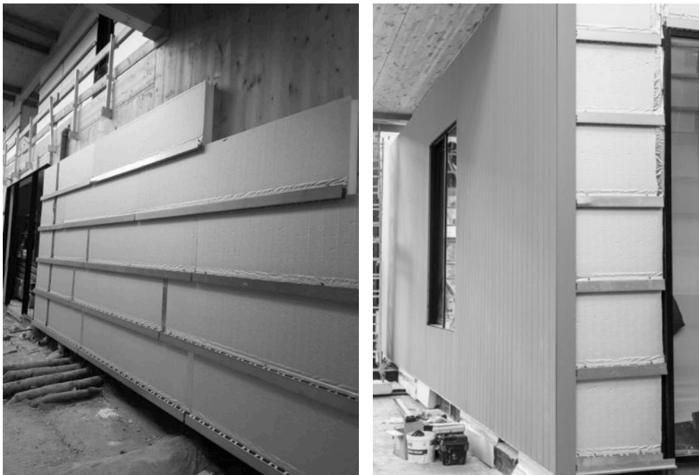
Figure 7: phases of installation of the facade build up
