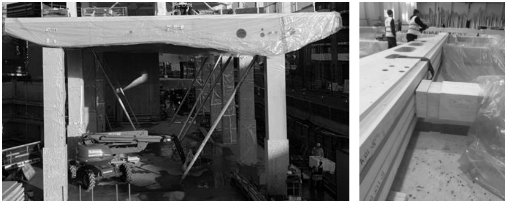
Figure 7: LVL beech beams and columns. LVL insertions.
