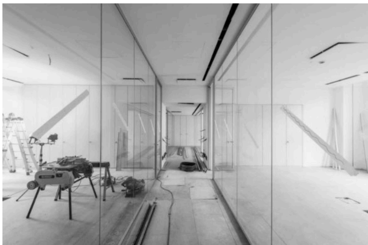
Figure 10: view of the internal finish
