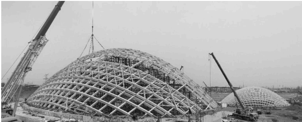
Figure 17: Medium Dome (foreground) and Small Dome (background) in Construction
