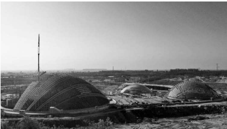
Figure 21: Current construction progress
