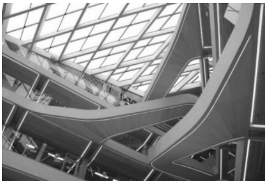
Figure 13. Main atrium stairs. Large span, helicoidal geometry, double curvature beams.
