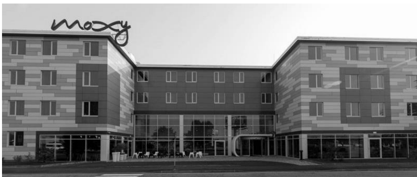
Figure 18: Moxy Hotel in Malpensa (VA)
