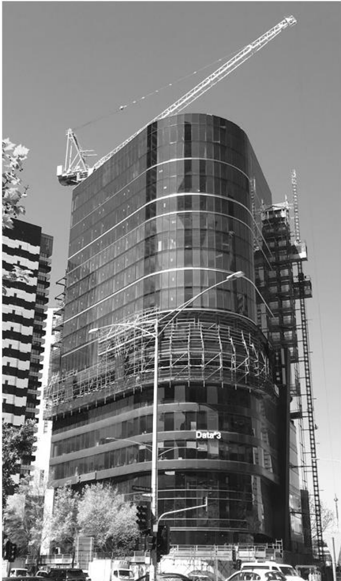
55 Southbank: A 10-storey CLT vertical extension during construction in Melbourne
