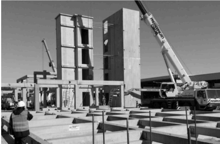
Figure 20: Concrete prefabricated structure
