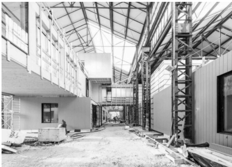
Figure 8: installation on site of the facade
