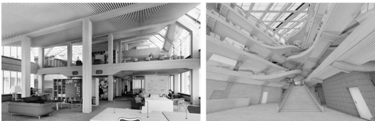
Figure 3: Interior with exposed timber structure (© Helen & Hard|Saaha)
