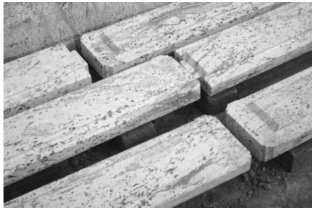
Figure 7: Door Frames, Chennai House
