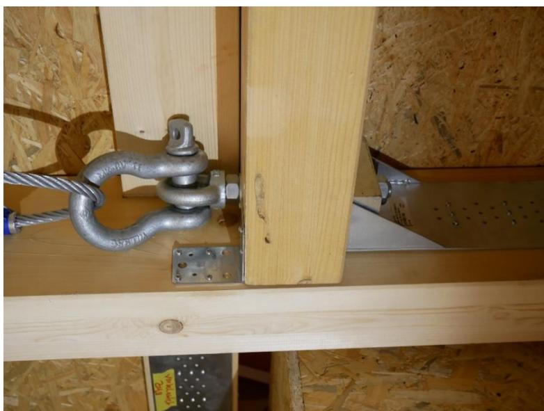
Figure 8: Anchorage on floor slab to pull on the building.
