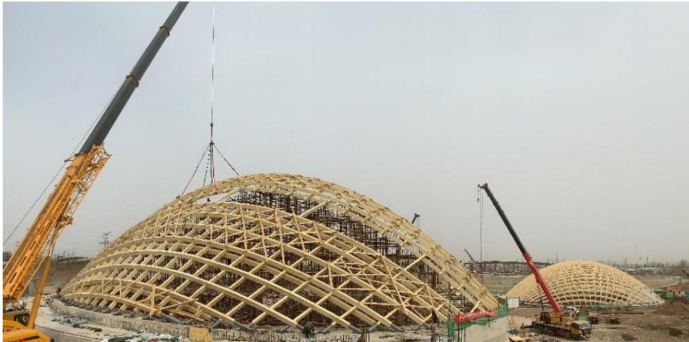
Figure 17: Medium Dome (foreground) and Small Dome (background) in Construction
