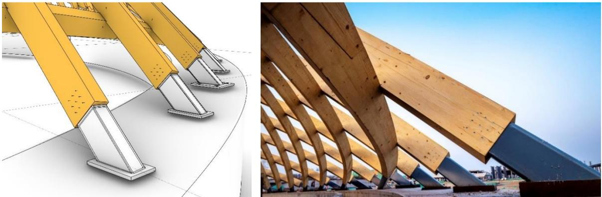
Figure 6: 3D model and Completed Base Connections
