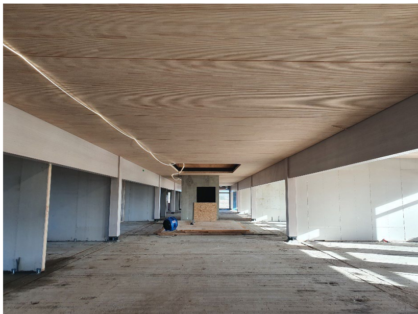
Figure 9: TSBOne, state of the art skeleton structure with 10 m clear span, Aarhus, Denmark
