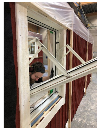
Figure 3: Attaching insulation and sealing in vertical window installation.
