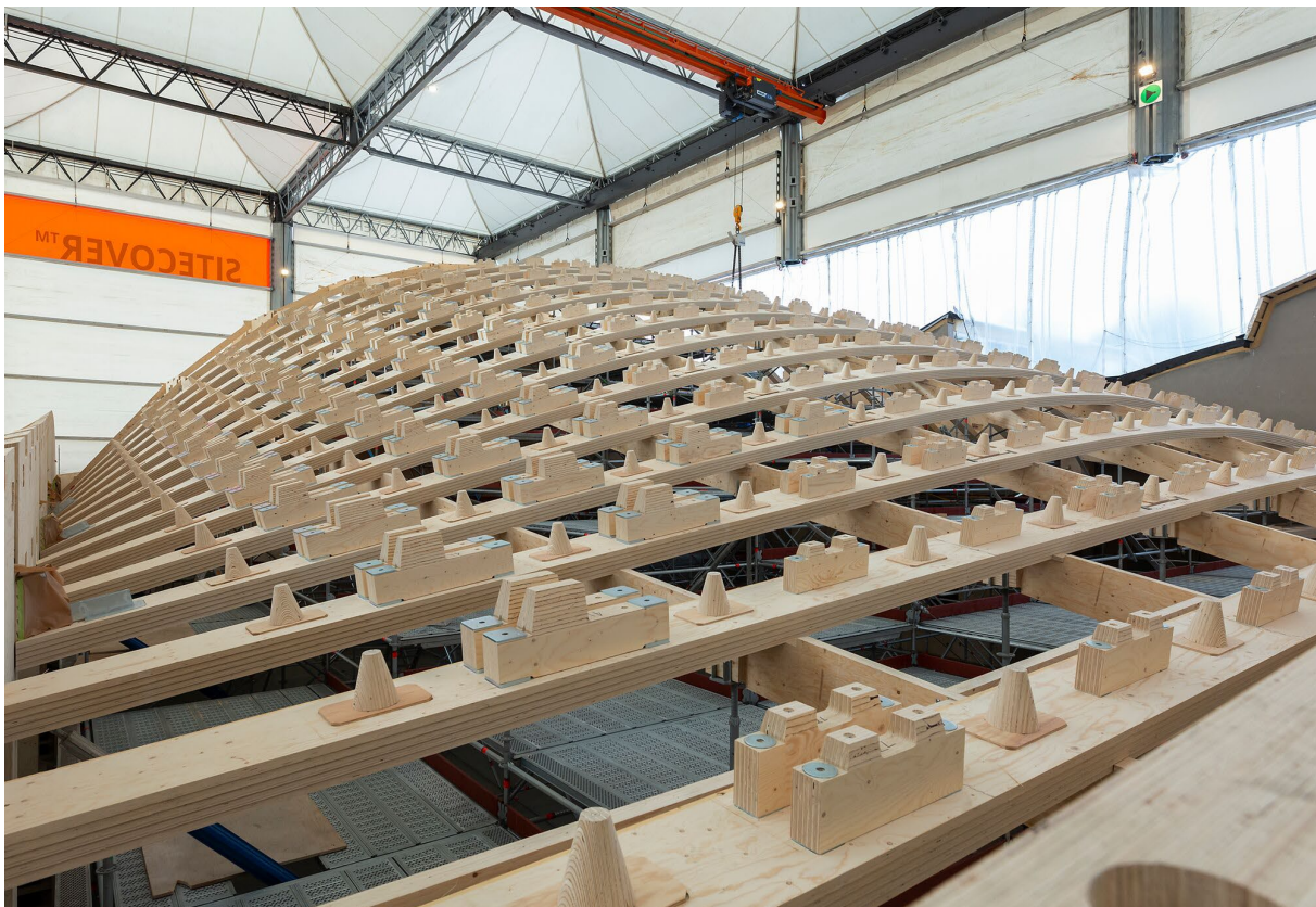
Figure 4/ Installation grid shell roof with dowelled girders / National Museum of Science and Technology
