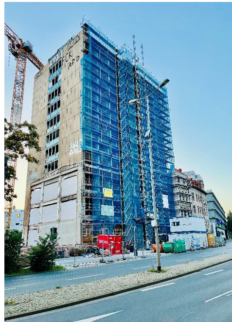
Figure 1: Industrial high-rise building being redesigned for modern flats, in Erfurt, Germany
