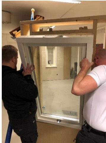
Figure 17: Placing a window into the window opening.
