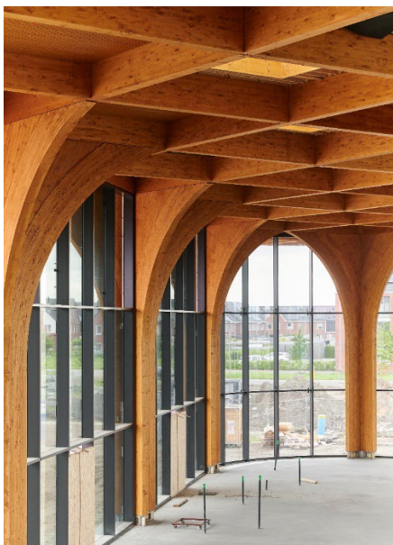
Picture 5: Diagonal grid of cross-shaped curved trusses
