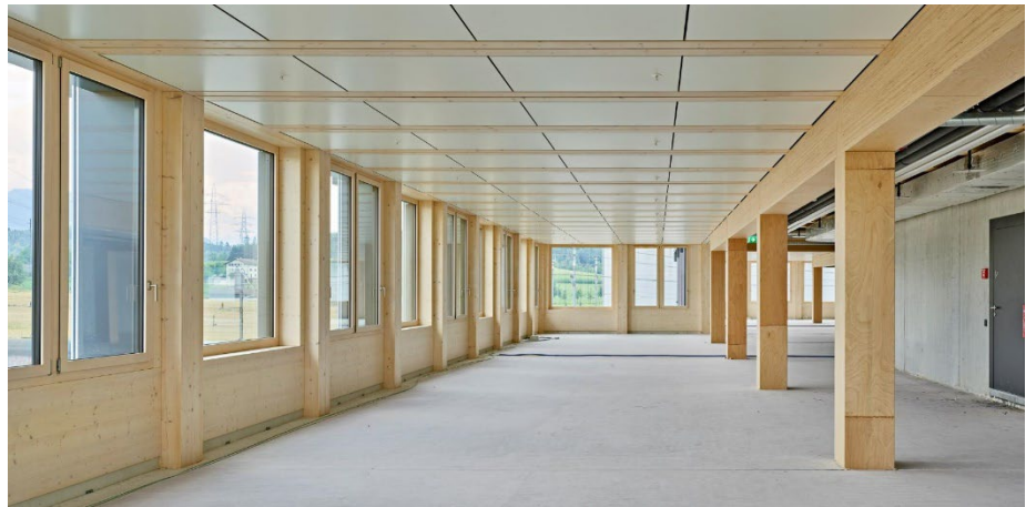
Figure 3: Timber skeleton frame from BauBuche GL75
