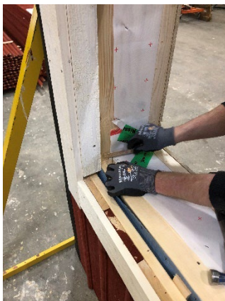
Figure 1: Preparations for direct vertical window installation.
