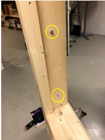
Figure 16: Click-In screws in window opening (marked yellow).
