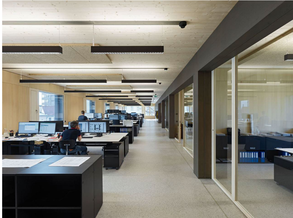
Figure 8: Skeleton structure from BauBuche posts and beams with CLT floors
