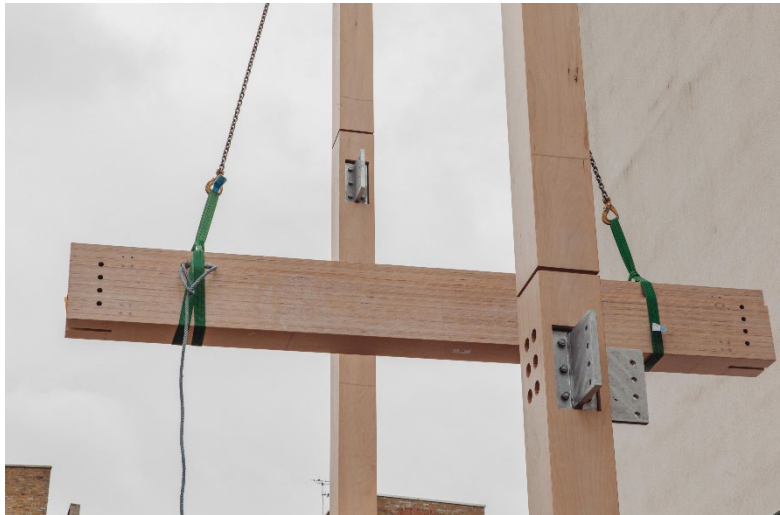
Figure 11: Connection detail, Black and White Building, London
