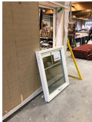
Figure 2: Window about to be installed vertically.
