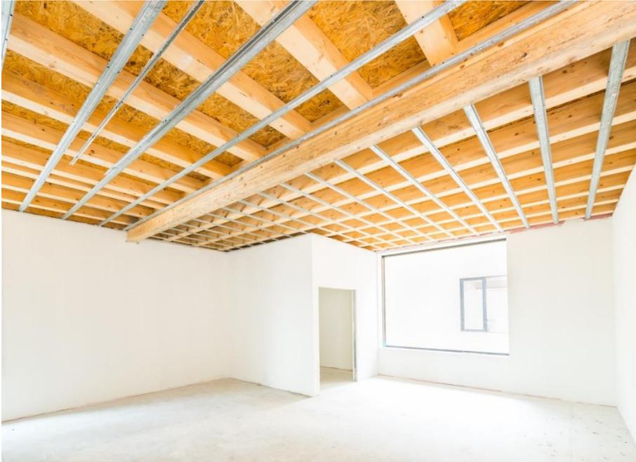
Figure 9: internal view of the spaces with plasterboard walls and the counter ceiling ready to be put in place
