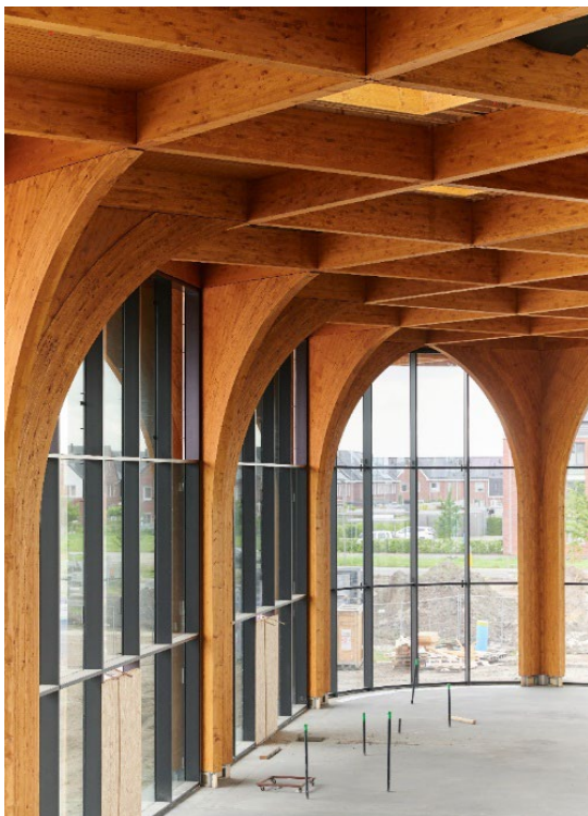
Picture 5: Diagonal grid of cross-shaped curved trusses
