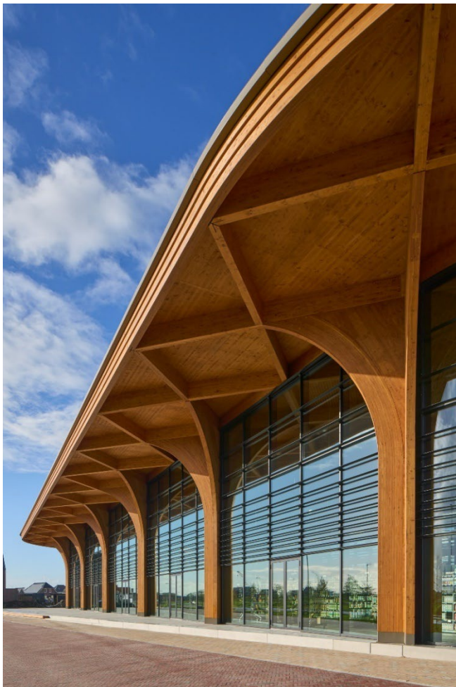
Picture 3: Side view wooden construction and transparent facade
