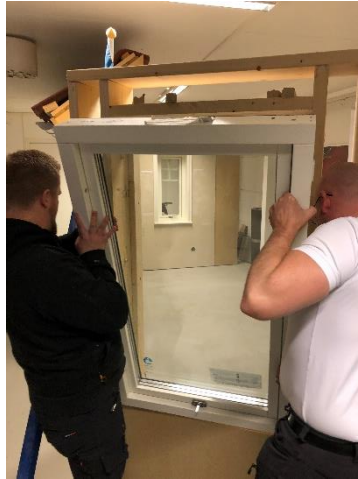
Figure 17: Placing a window into the window opening.
