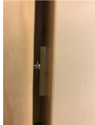
Figure 18: Click-In snap joint glided over the screw head and the fixture system is spring-closed.
