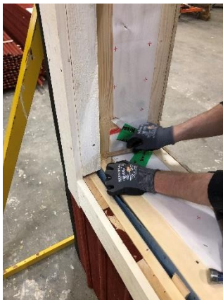
Figure 1: Preparations for direct vertical window installation.
