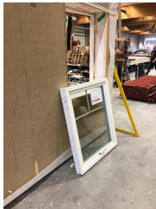
Figure 2: Window about to be installed vertically.
