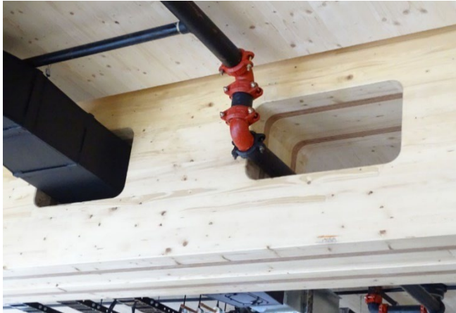
ip and Figure 4: View of large rectangular holes with internal beech LVL reinforcement plates at the International House Sydney
