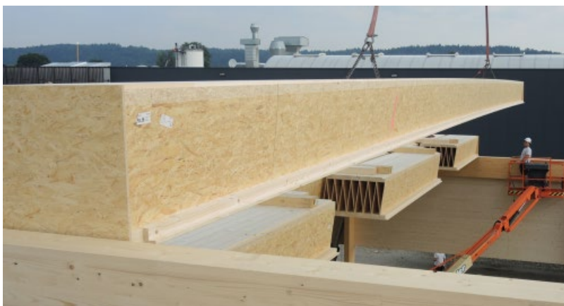
Figure 9: Mounting of Kielsteg elements with a length of 23 m at a building site. The also shown elements with shorter lengths enable roof windows
