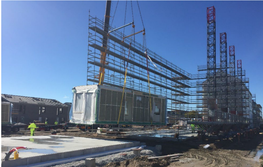
Figure 6: Wood-based volumetric elements are assembled fast on the building site
