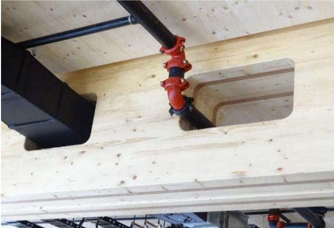
ip and Figure 4: View of large rectangular holes with internal beech LVL reinforcement plates at the International House Sydney
