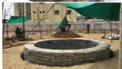
Well Building | Well Sinking
