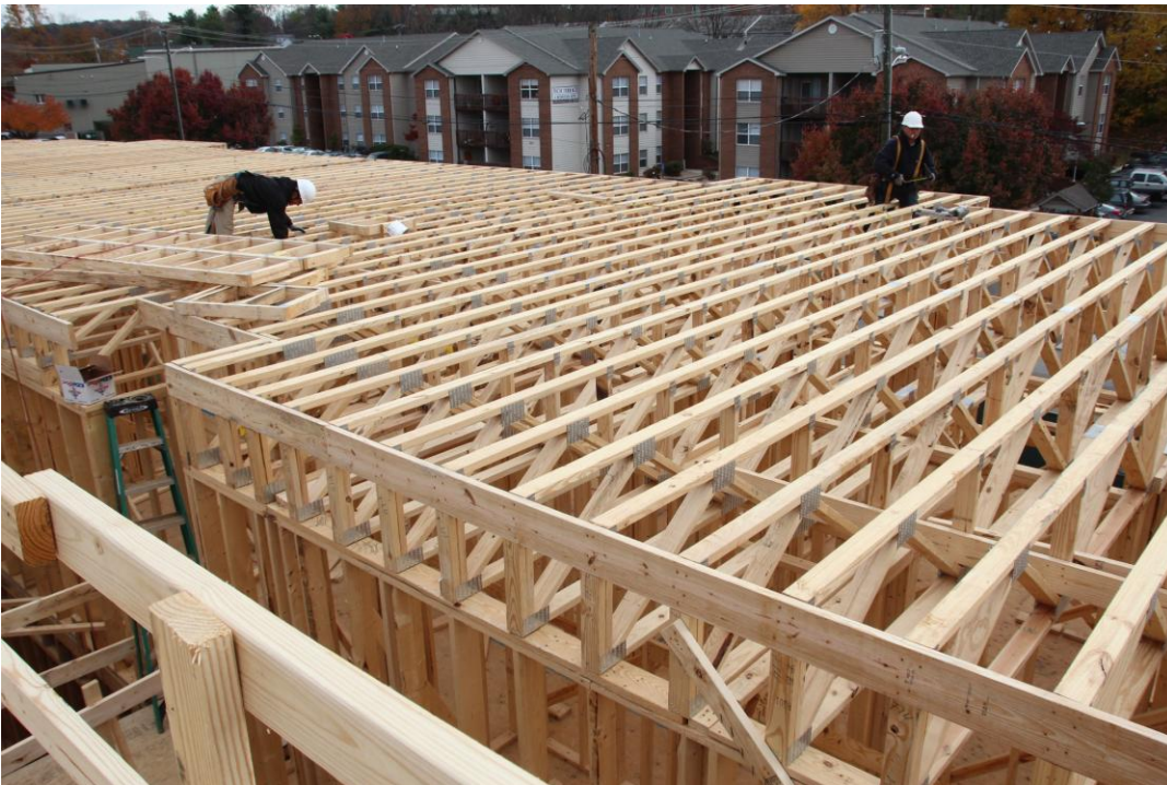
Figure 4: Metal plate connected wood floor trusses being installed.
