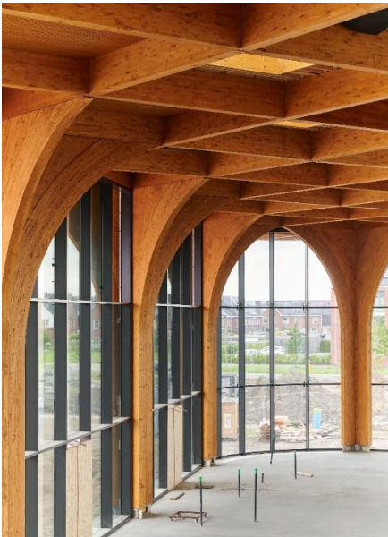
Picture 5: Diagonal grid of cross-shaped curved trusses
