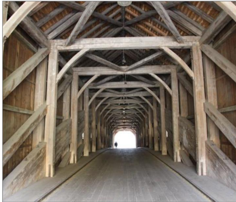
20 Wintersey teeth beam wood bridge in Switzerland Hasle Rüggsau, 1839
