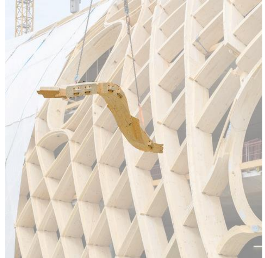
15 Complex construction from preformed glulam beams
