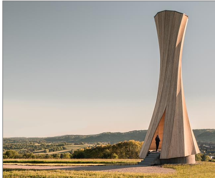
14 Construction from hygroscopic preformed elements
