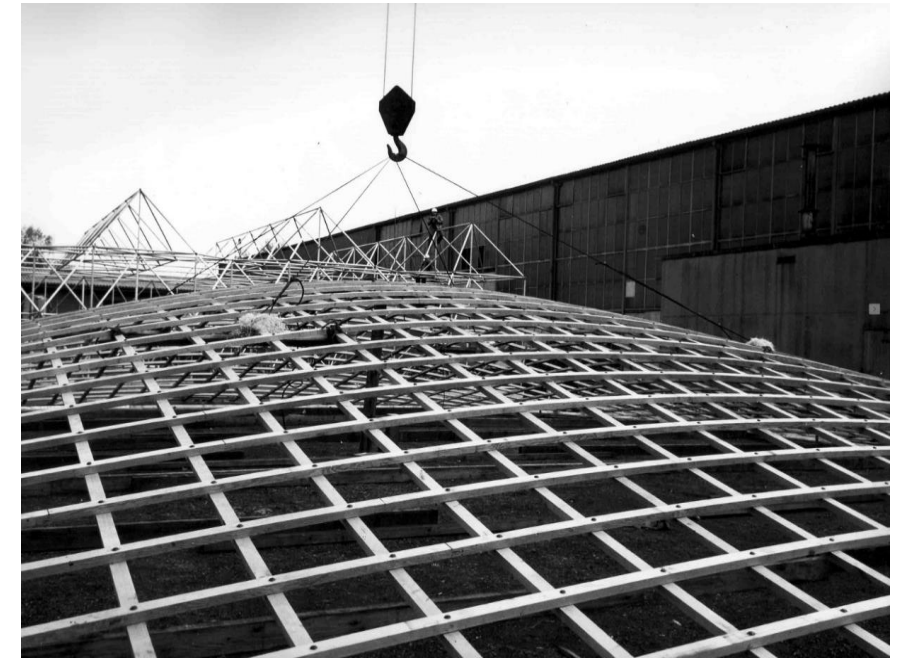
17 Grid shell construction, step 2: onsite forming process
