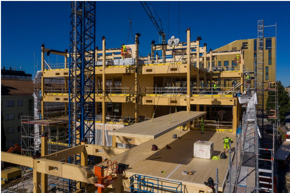
Figure 19: Construction site. Photography: Gustav Kaiser
