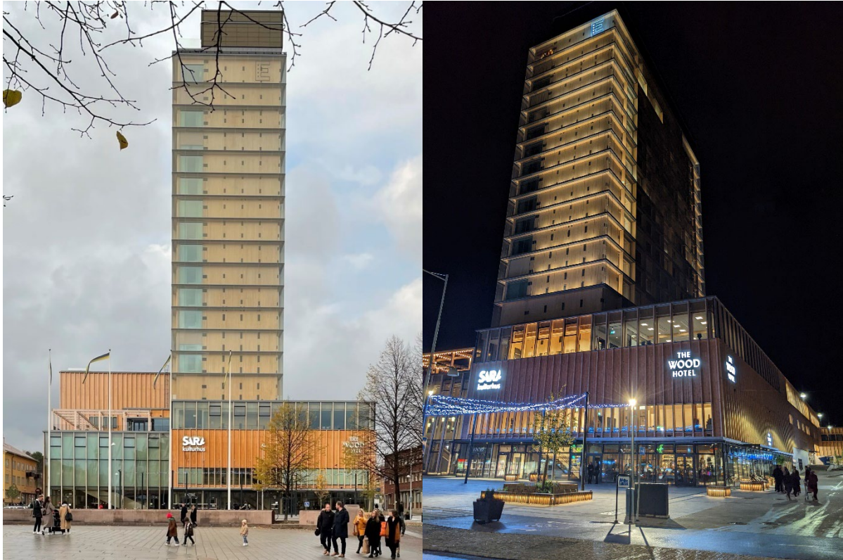
Figure 1: Main entrance and hotel complex on a grey day and at night. Photo by Brian Perktold, Mark Wojcik
