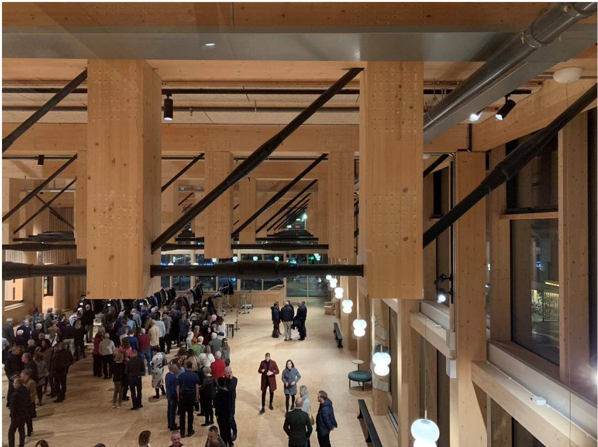
Figure 10: Hybrid trusses over lobby area. Photo by Mark Wojcik
