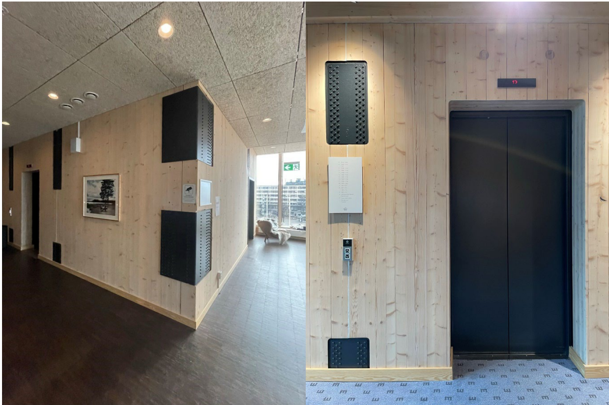
Figure 7: Black plates connecting main core CLT panels. Photo by Mark Wojcik
