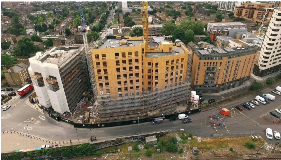
Image 5: Dalston Lane - under construction
