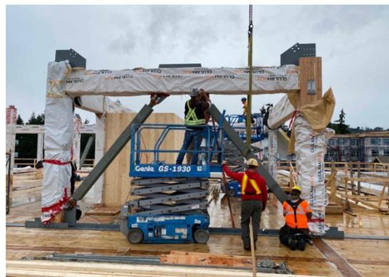
Figure 6: Terminus Brace Frame During Construction
