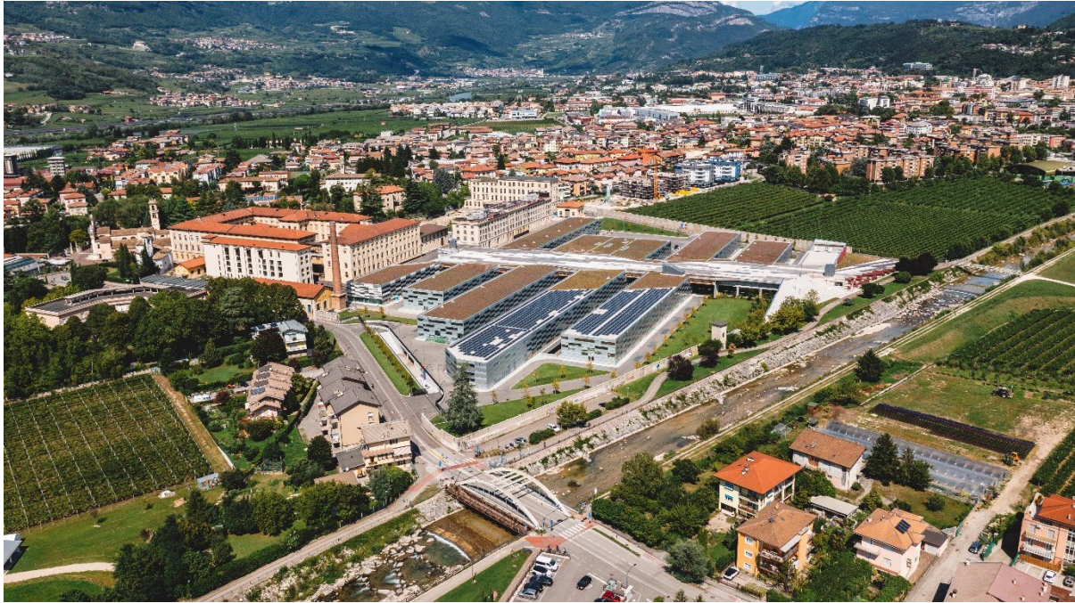
Picture 5: The structures as they appear now, a little more than two years after the start of the construction site works (courtesy Trentino Sviluppo S.p.A.).
