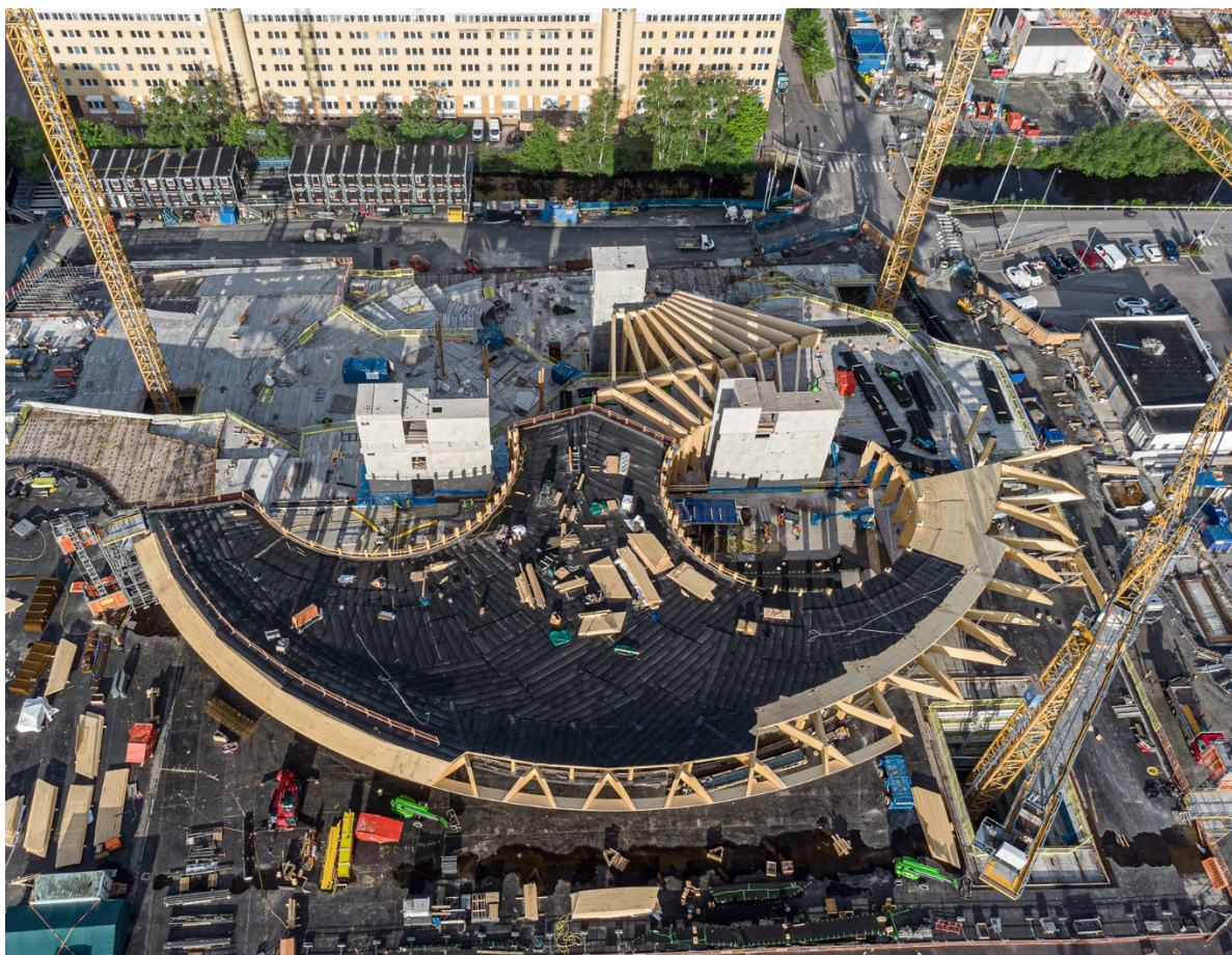
Picture 14: Birdsvie during installation of timber structure
