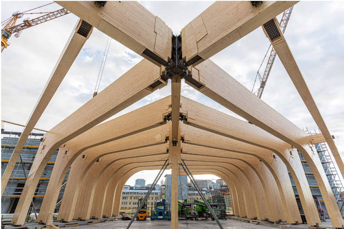
Picture 11: Cover plates around star node
