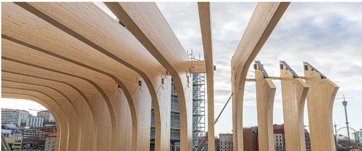
Picture 8: Curved corner connection during installation
