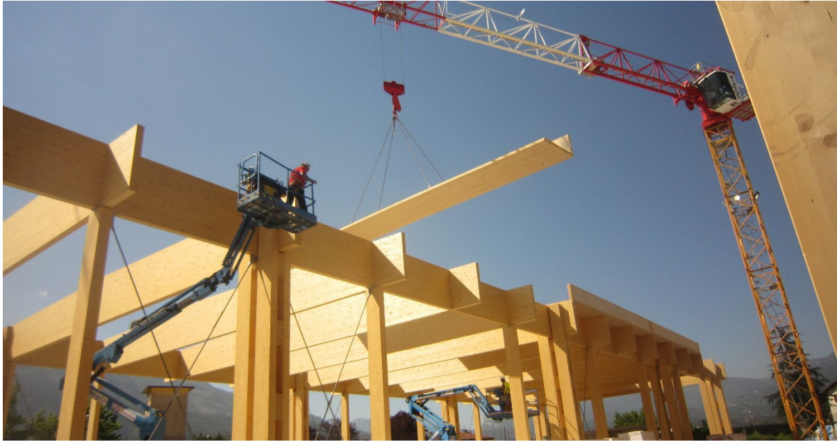
Picture 14: Placing of the CLT edge panel with the factory pre-assembled moulding
