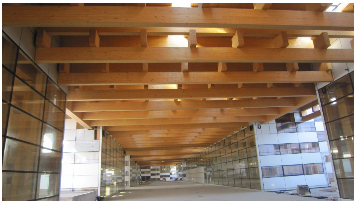
Picture 11: The tunnel that interconnects the buildings
