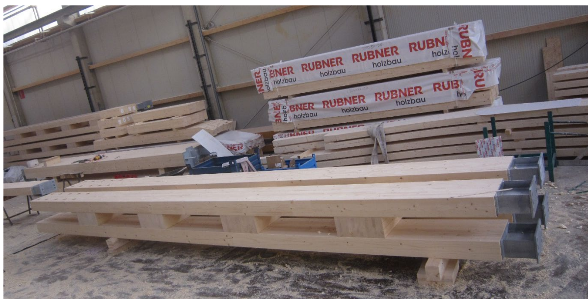
Picture 13: Pre-assembly of the columns at the production plant
