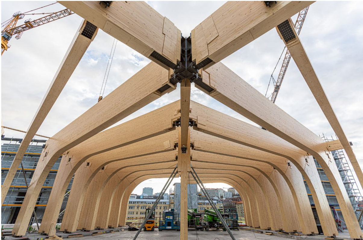
Picture 11: Cover plates around star node
