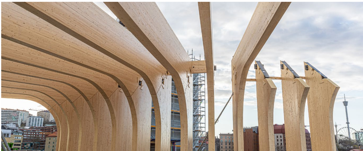
Picture 8: Curved corner connection during installation
