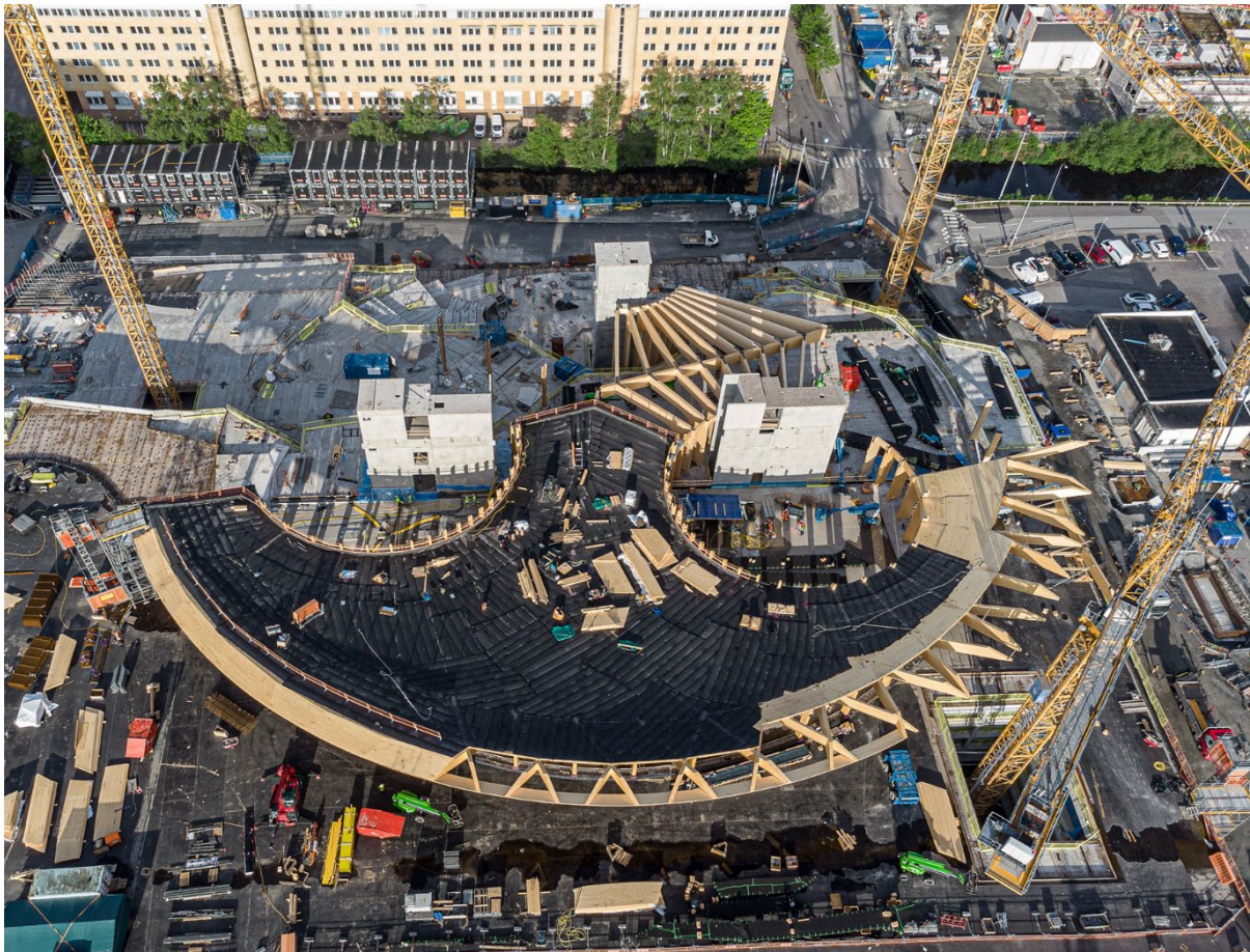
Picture 14: Birdsview during installation of timber structure
