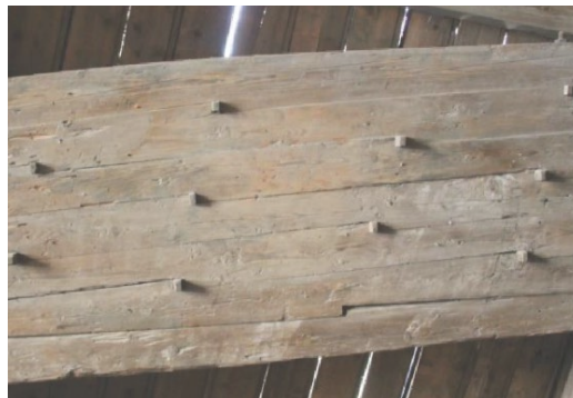
Figure 10: Tooth-beam at the Wintersey-bridge
