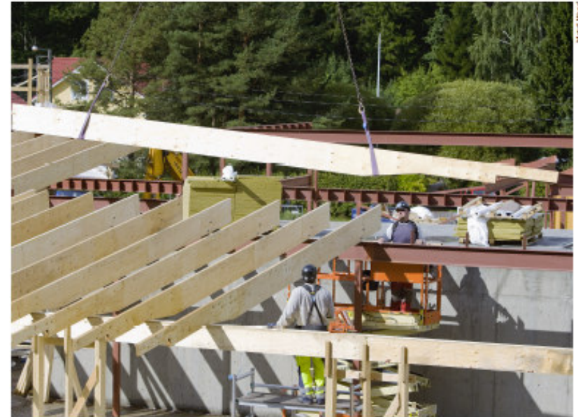
Figure 1.49. LVL-P roof beam cut to special shape.
