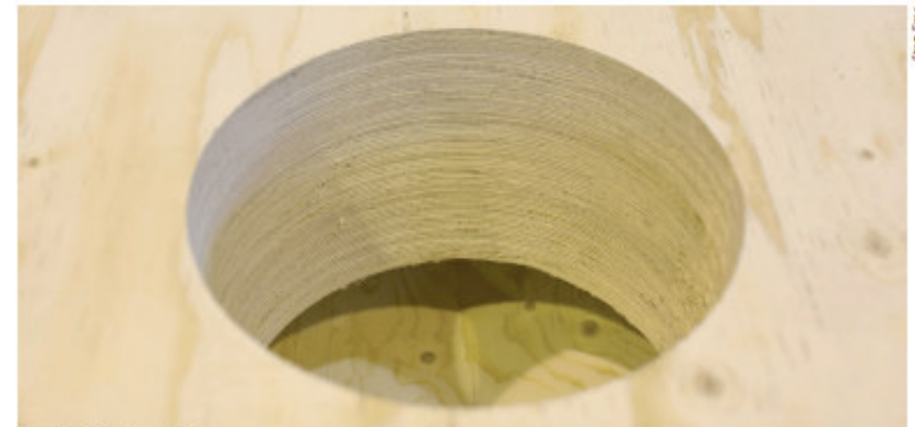
Figure 1.50. Hole in an LVL beam.
