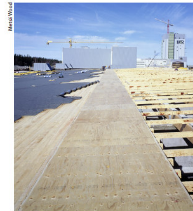
Figure 1.4 LVL-C roof panels.
