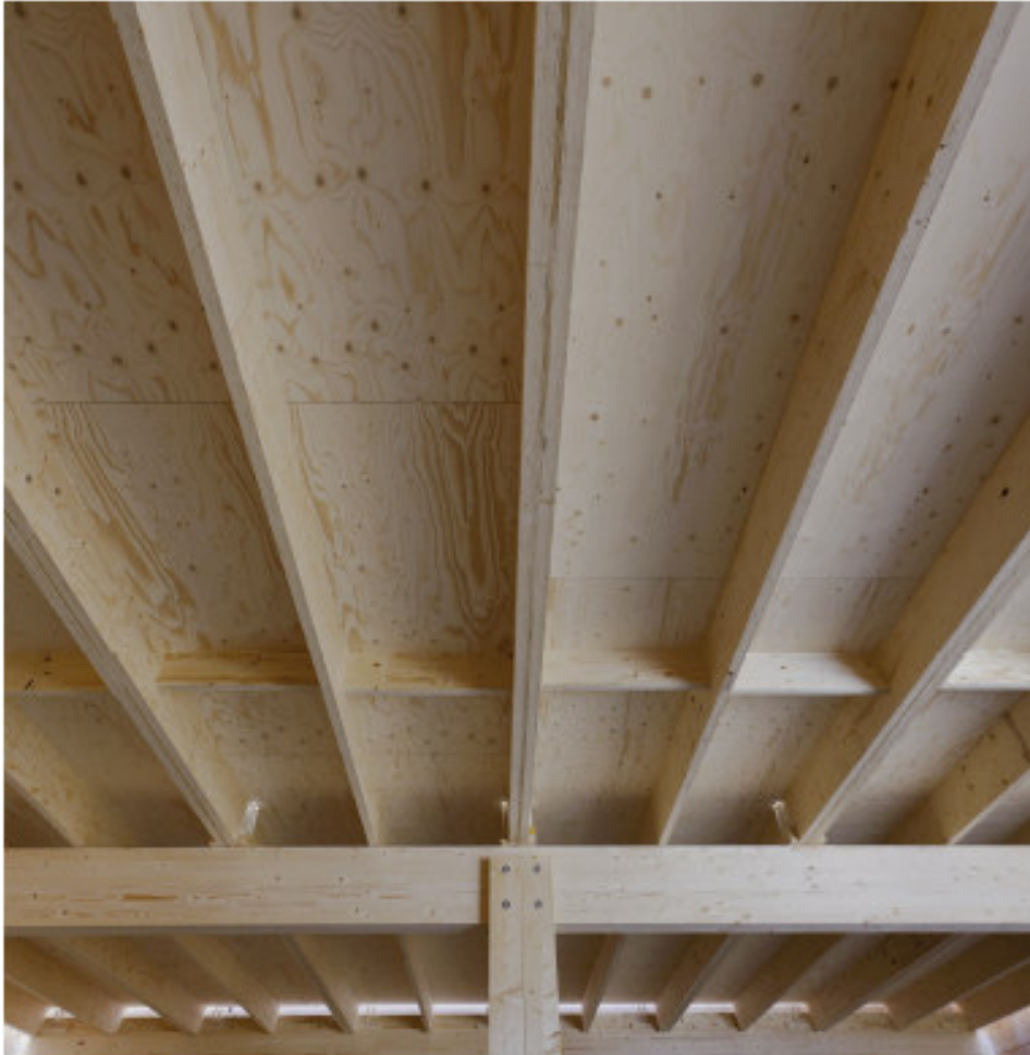
Figure 1.1 LVL roof structure, K-Rajamarkat, Utsjoki, Finland.
