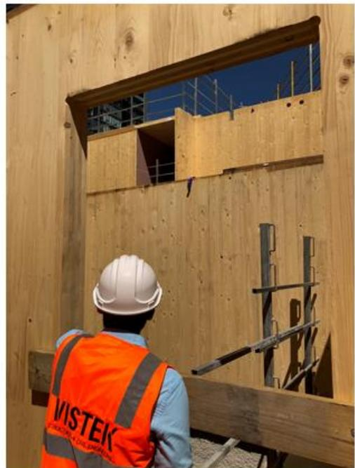
55 outhbank: A 10-storey CLT vertical extension during construction in Melbourne
