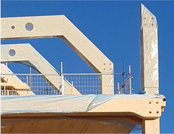
Figure 8: On site picture. Direct timber connection
