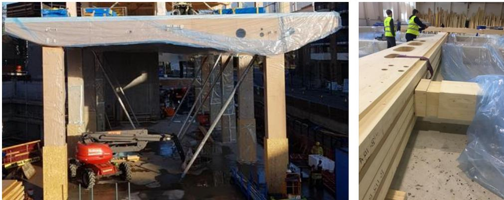
Figure 7: LVL beech beams and columns. LVL insertions.
