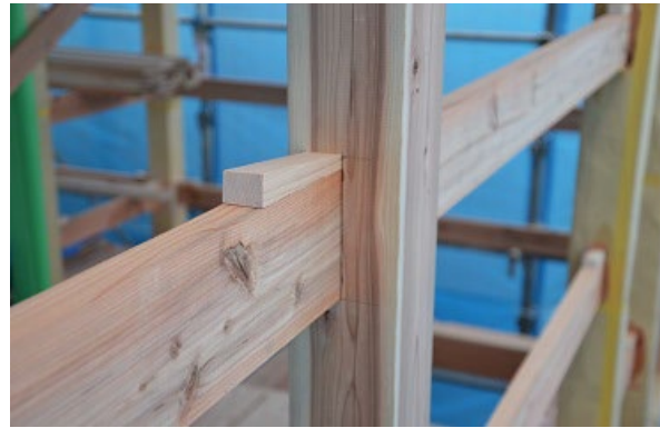
Post 120 mm x 120 mm with a nuki and a wedge
