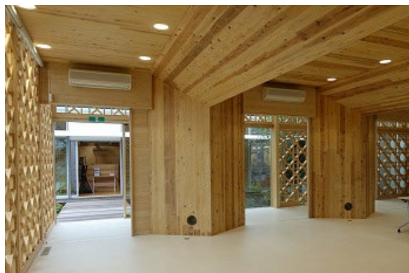
V-shaped beams of CLT
