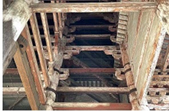
Interior of Namdai-mon: nukis run through columns.
