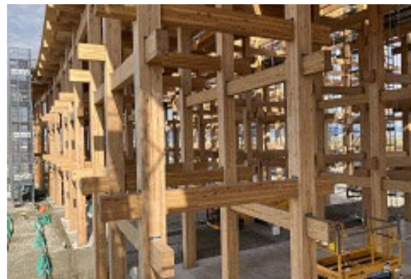
under construction Details of the nuki connection (courtesy of Obayashi Corporation)
