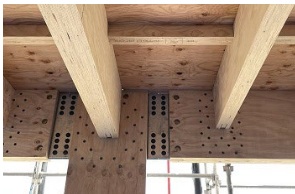
Example of rigid connection: designed by architectural design office Building Landscape in 2023
