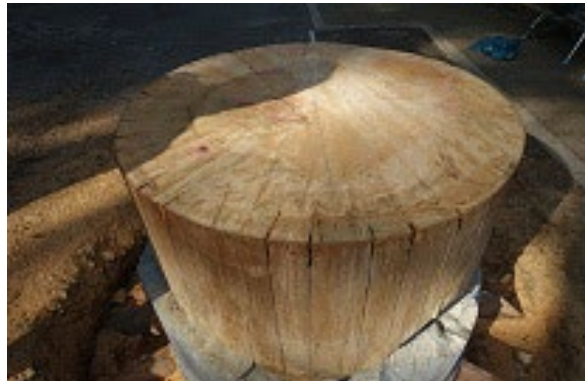
Cross-section of one of the pillars – 1067 mm in diameter
