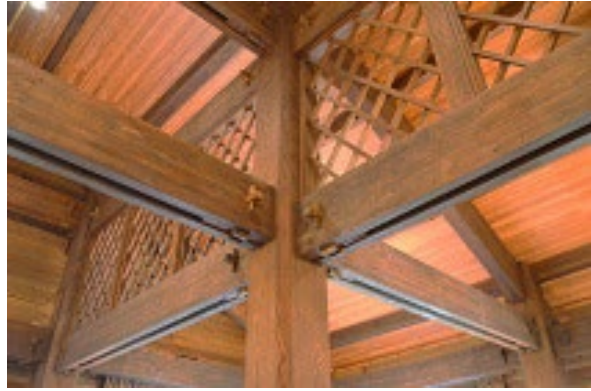
Hakkoda Hotel: 1991 designed by Masao Hayakawa Modernized four-way insert construction ( Kanzashi )
