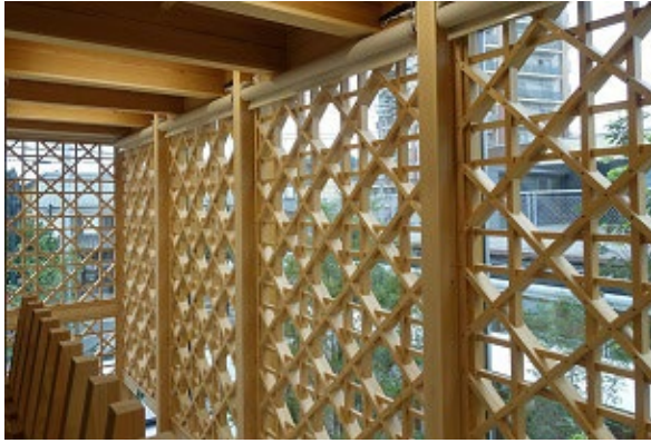
shear walls against lateral forces transmitting light
