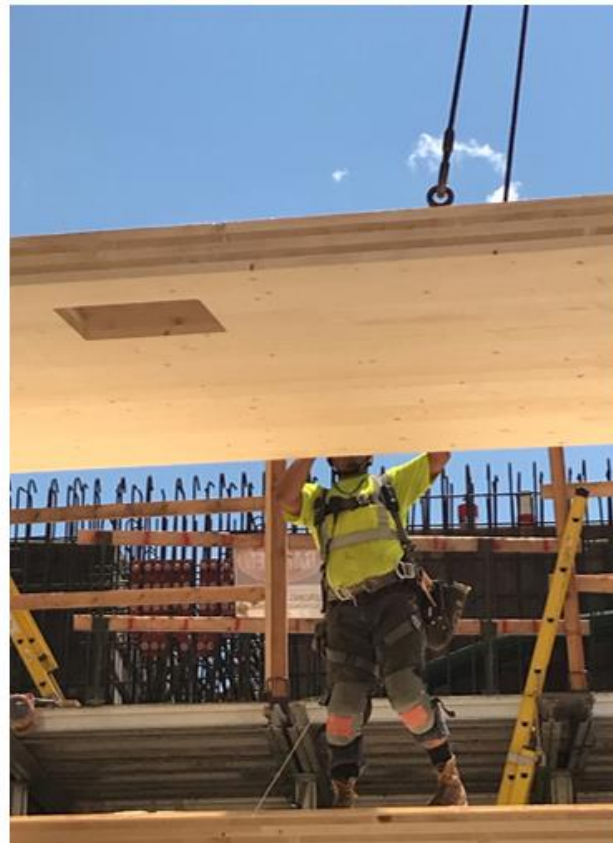
CLT was pre-cut for column penetrations
