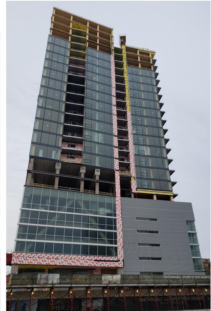
Level 26 (Roof) Topped Out (December 2021)
