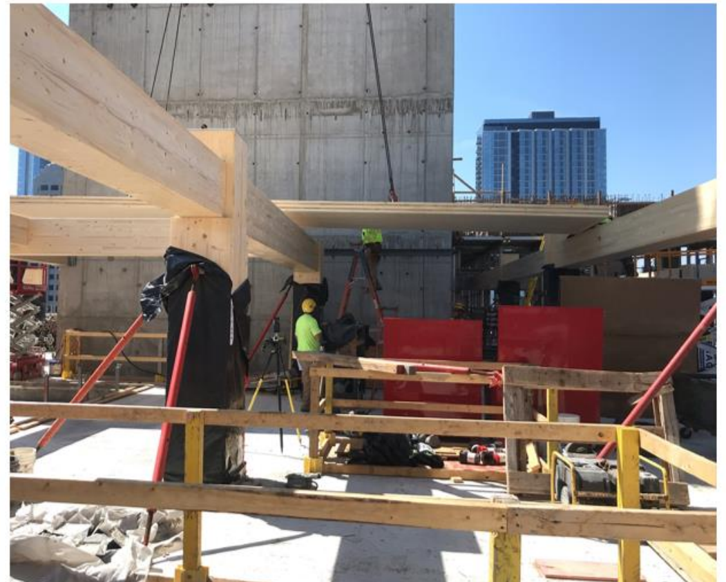
CLT installation at concrete core
