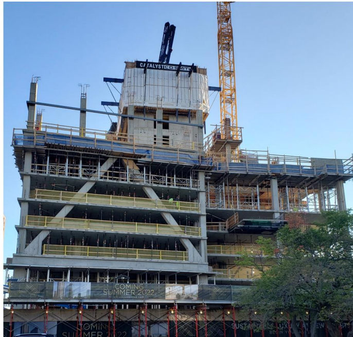
Start of Timber Construction (June 2021)
