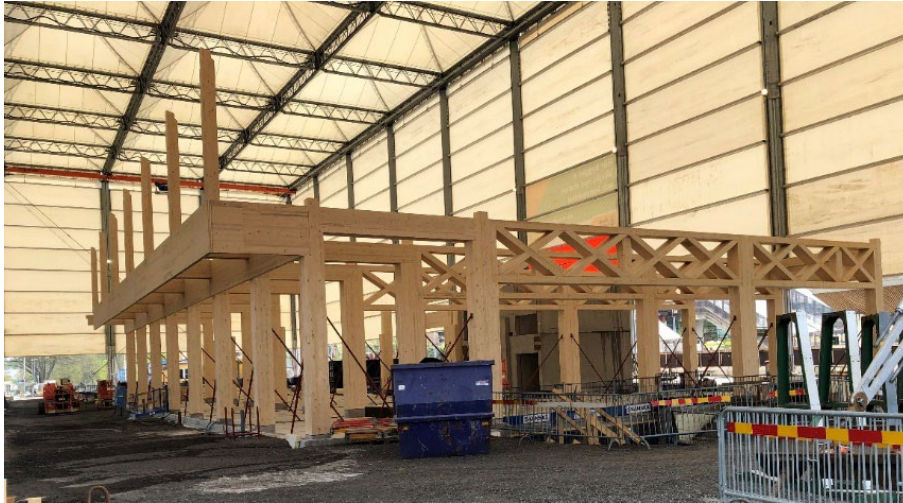
Figure 6: Photo showing structural members in timber and concrete for the first floor of the building. Photo: Skanska
