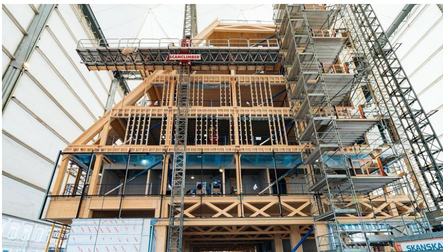
Figure 4: Photo during construction inside the construction site cover. Photo: Skanska
