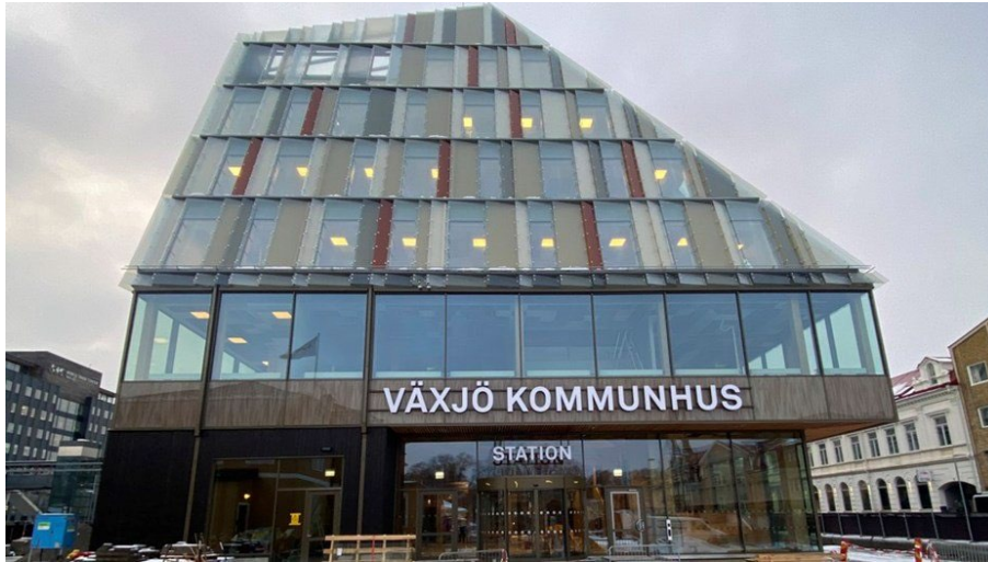
Figure 7: Photo of the exterior in the finished project in 2021. Photo: Skanska
