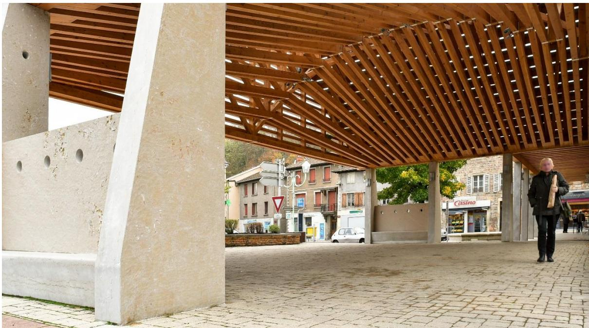
The Vinsobres childcare building, with massif wood structure, straw insulation and earth and lime plasters on the walls.
