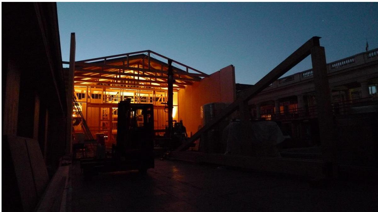
The fact of bringing prefabricated roof panels already waterproofed made it possible to advance each day by more than 120 m<sup>2</sup> (*hundred twenty squared meters*) covered and closed.
