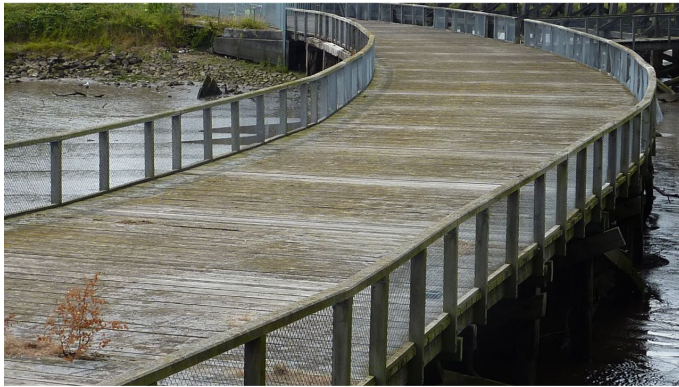
Figure 11: Lower Deck Lichen Growth
